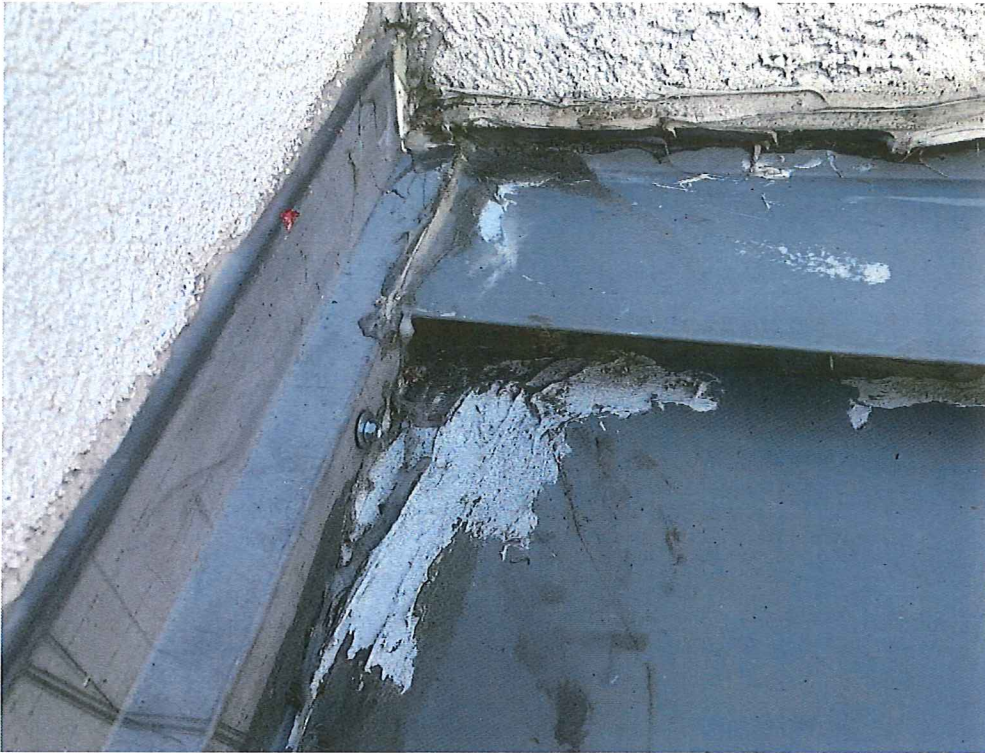
Photograph 9. Sealant applied at a sidewall - headwall termination joint.
