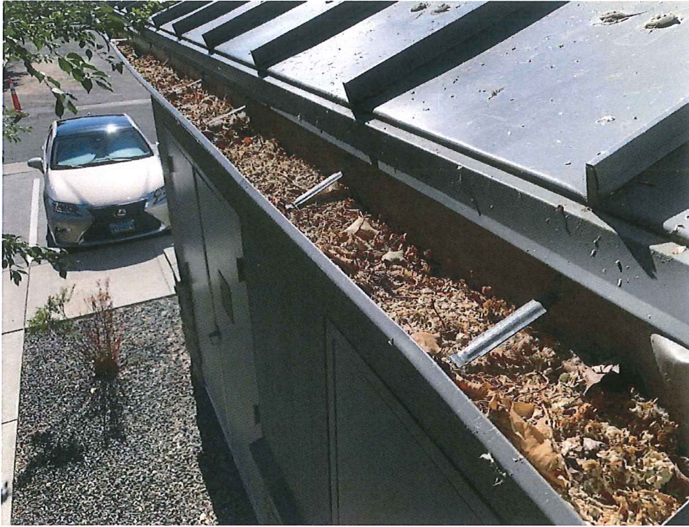
Photograph 13. Gutter filled with leaves.
