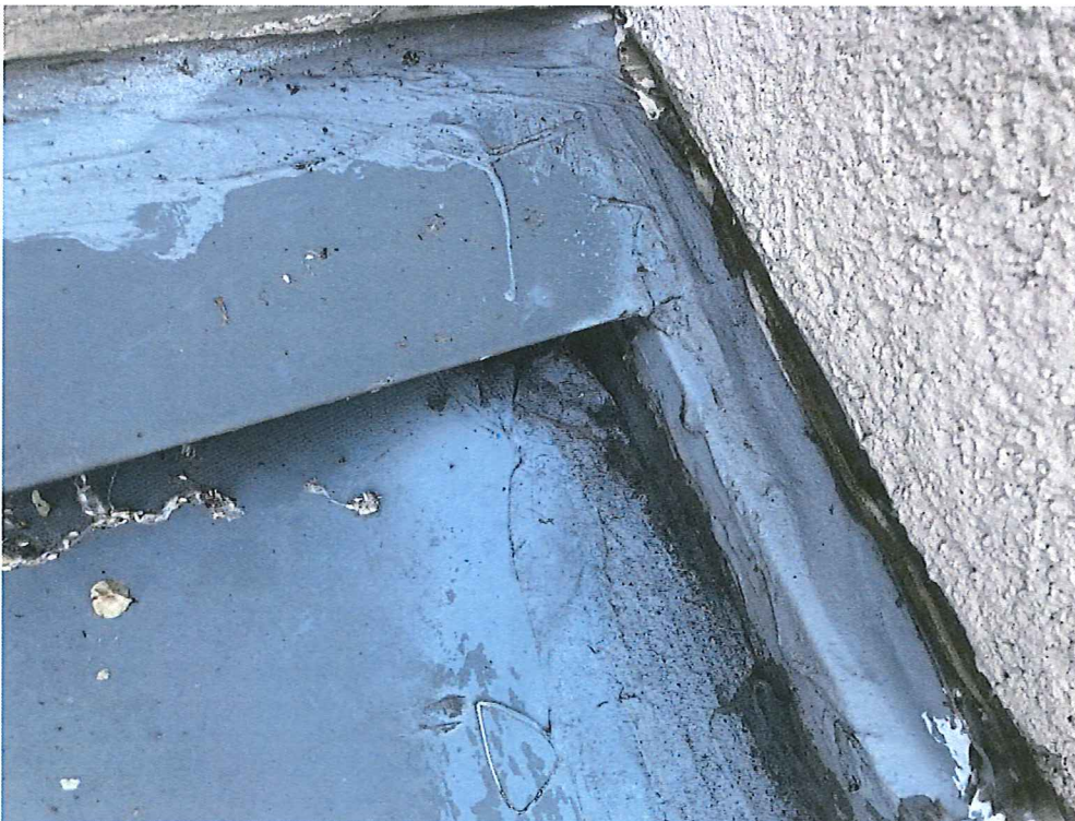
Photograph 10. Sealant applied at a sidewall - headwall termination joint
