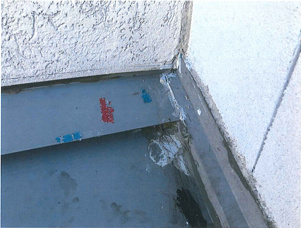
Photograph 7. Sealant applied at a headwall - sidewall termination joint.
