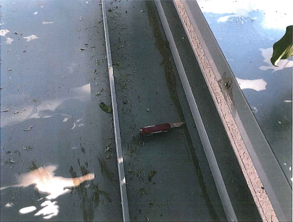
Photograph 12. Gap below the sidewall flashing.
