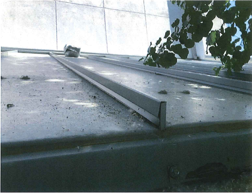
Photograph 3. Standing seam roofing as installed.
