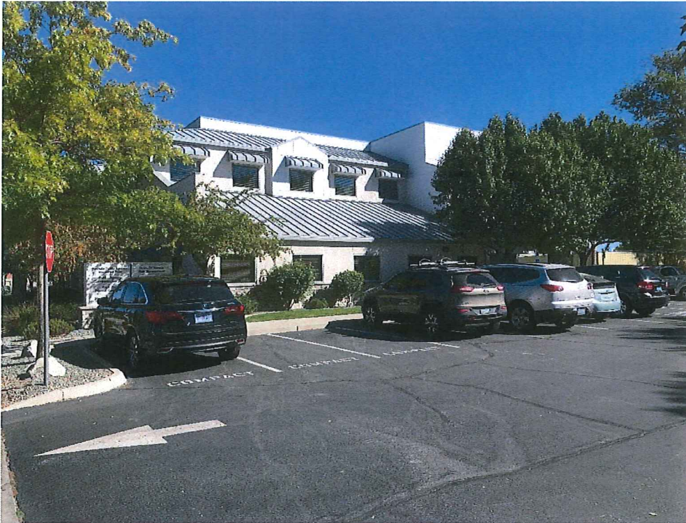
Photograph 1. View of the upper and lower roofs from the south.
