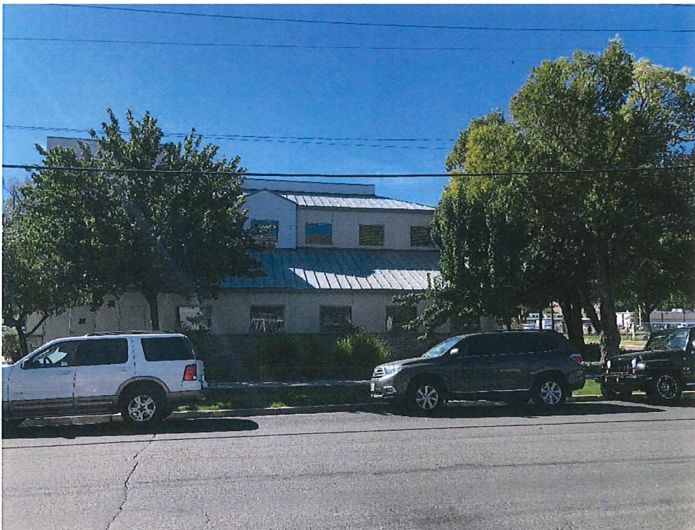
Photograph 2. View of the upper and lower roofs from the north.
