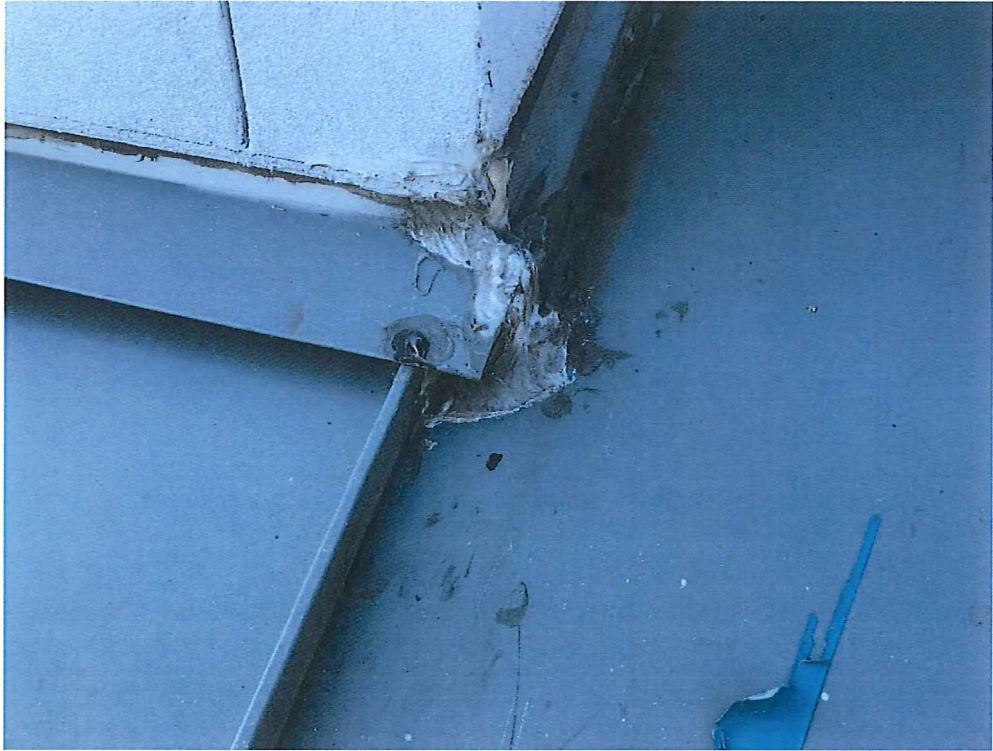
Photograph 8. Sealant applied at a headwall - sidewall termination joint.
