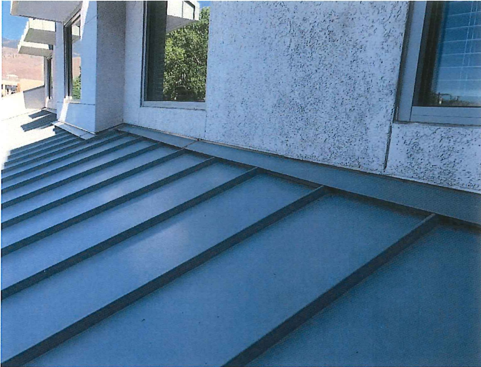
Photograph 5. Typical headwall termination flashing at the stucco wall.
