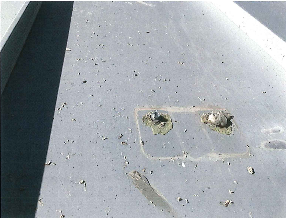
Photograph 4. Standing seam roofing with screws from a snow retention system.
